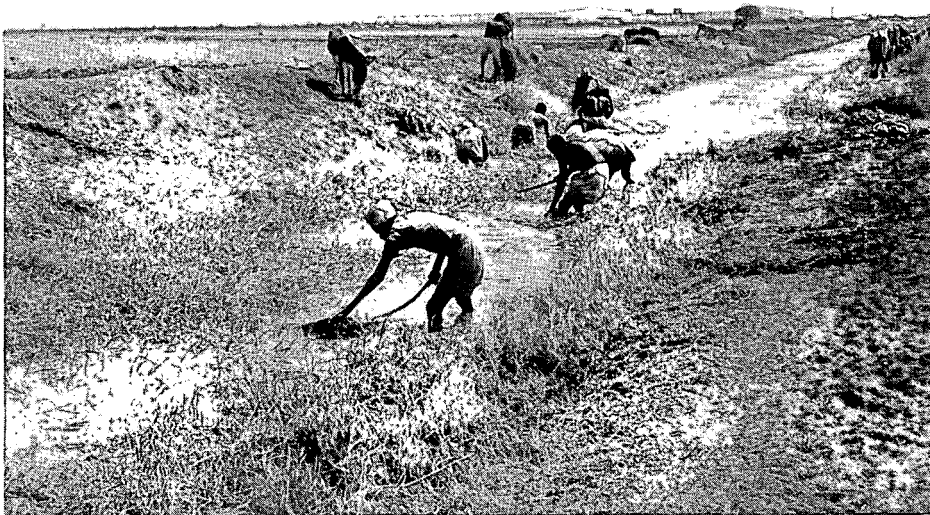
Figure 6.6 The manual removal of aquatic weeds in irrigation canals is usually the only economically feasible method in tropical countries
